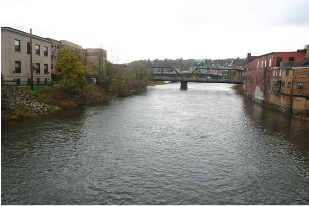
Fig 3a. Lower Oil Creek looking downstream. Patched hole in brick building can be seen on the right.
