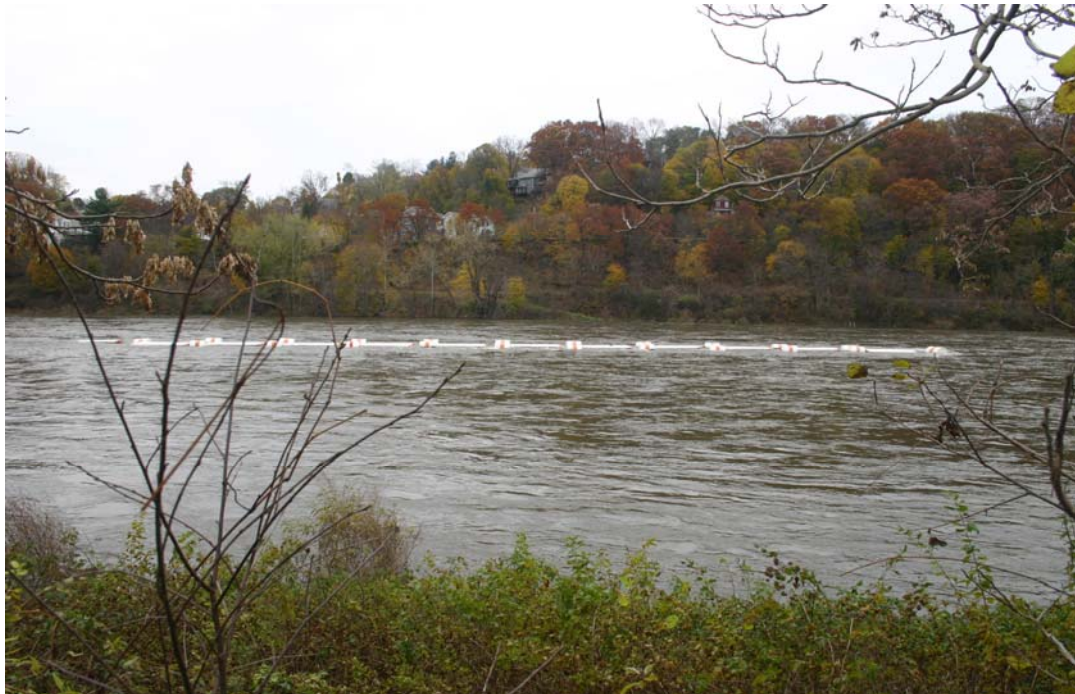
Fig. 6. Allegheny River Ice Boom spans trailing in the current from the central anchor. Spans are pulled to shore and anchored to the banks.
